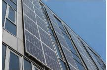
a vertical placement, also allows you to utilize more panels. This layout means you can install more panels at a lower cost. You'll recoup the expense quickly since you have more panels soaking up sun light." [https://solvoltaics.com/solar-panels-vertical-or-horizontal/]
